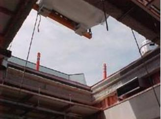
Exam room with magnet delivery through the roof
