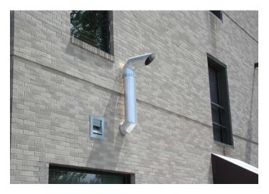
Typical side wall exterior vent exit
