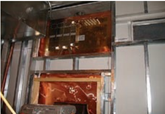
Electrical Filters/Med Gas/Sprinkler line
