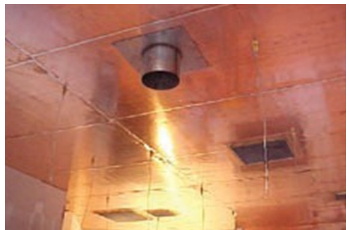
Cryogen vent at RF Shield
