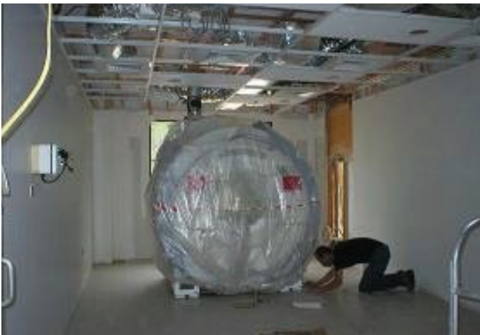
Exam room with magnet delivery through the wall.
