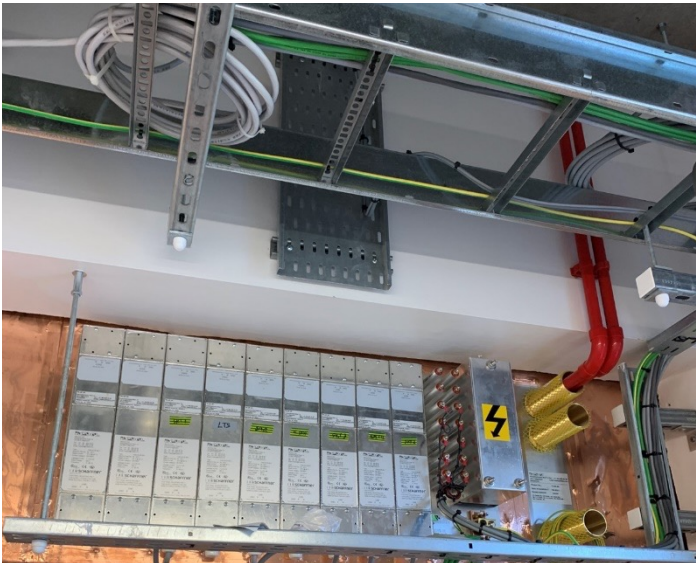
Penetration Panel Filters and Wave Guides
