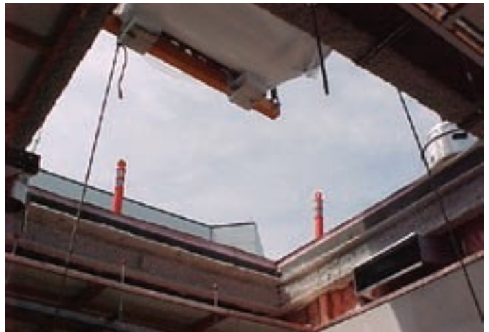
Exam room with magnet delivery through the roof.
