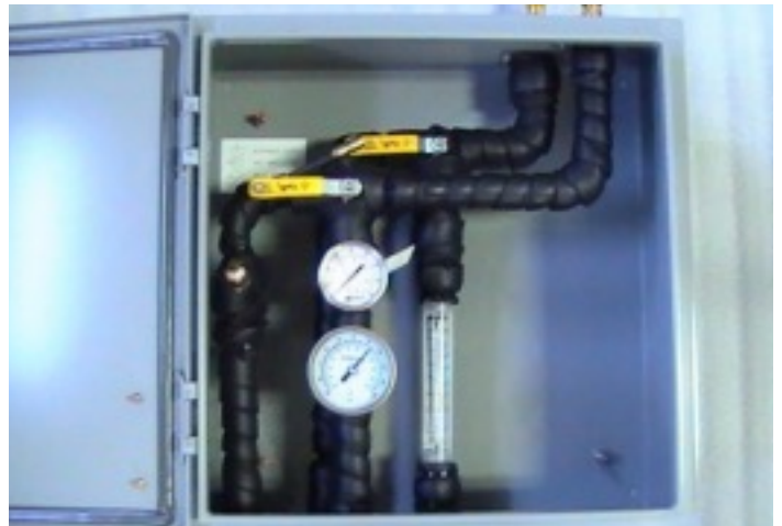
Chiller Water Bypass System
