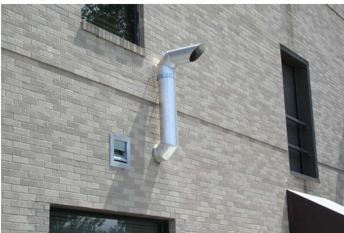
Typical side wall exterior vent exit
