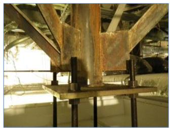
Figure 46 - Above Ceiling Cable Management Support
