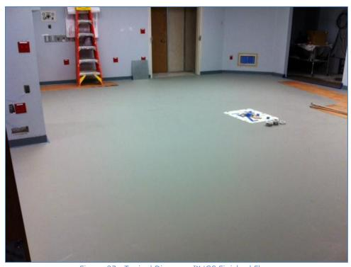
Figure 23 - Typical Discovery™ IGS Finished Floor
