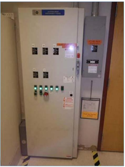
Figure 22 - Innova Main Disconnect Panel
