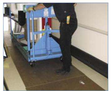
Figure 17 - Masonite Board Floor Protection
