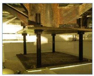
Figure 47 - Adjustable Cable Management Support Plate
