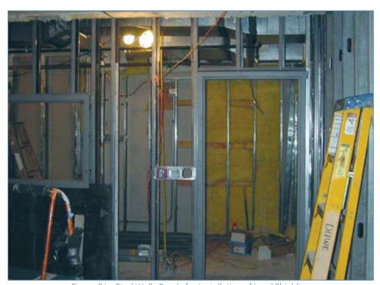
Figure 24 - Stud Walls Ready for Installation of Lead Shielding
