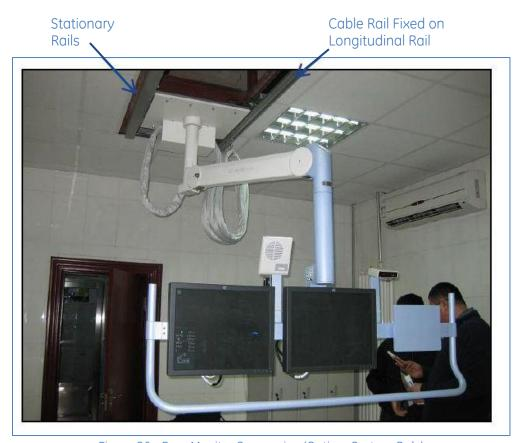
Figure 26 - Ergo Monitor Suspension (Optima System Only)
